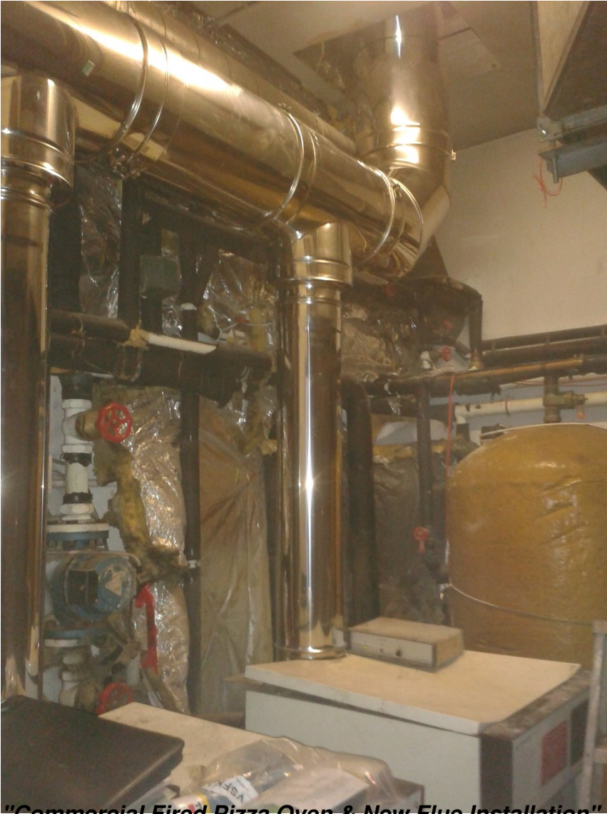
"Commercial Fired Pizza Oven & New Flue Installation"
