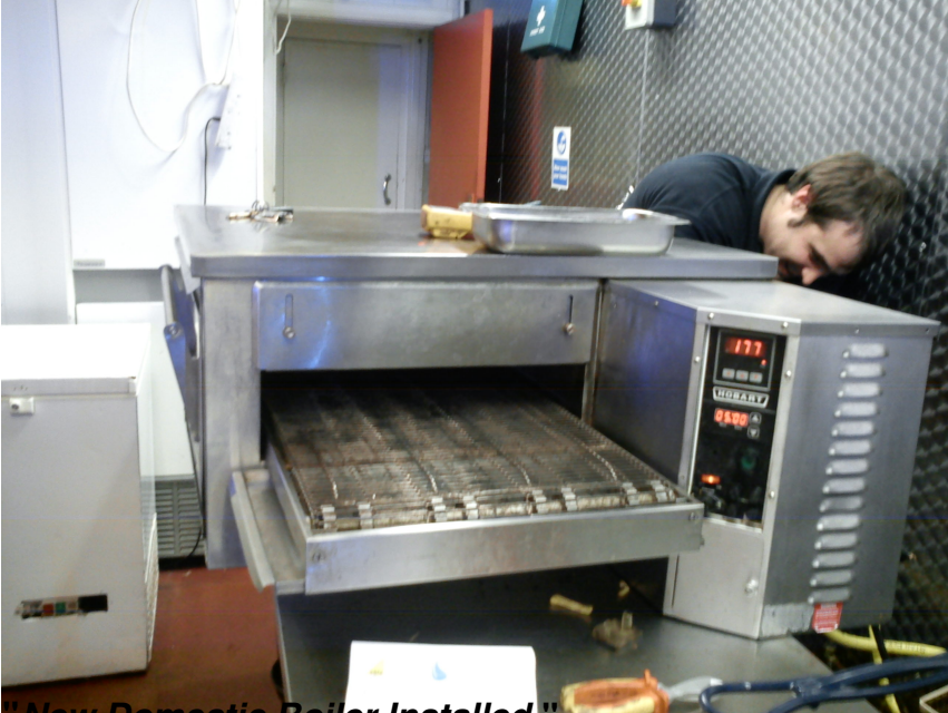
New Domestic Boiler Installed
